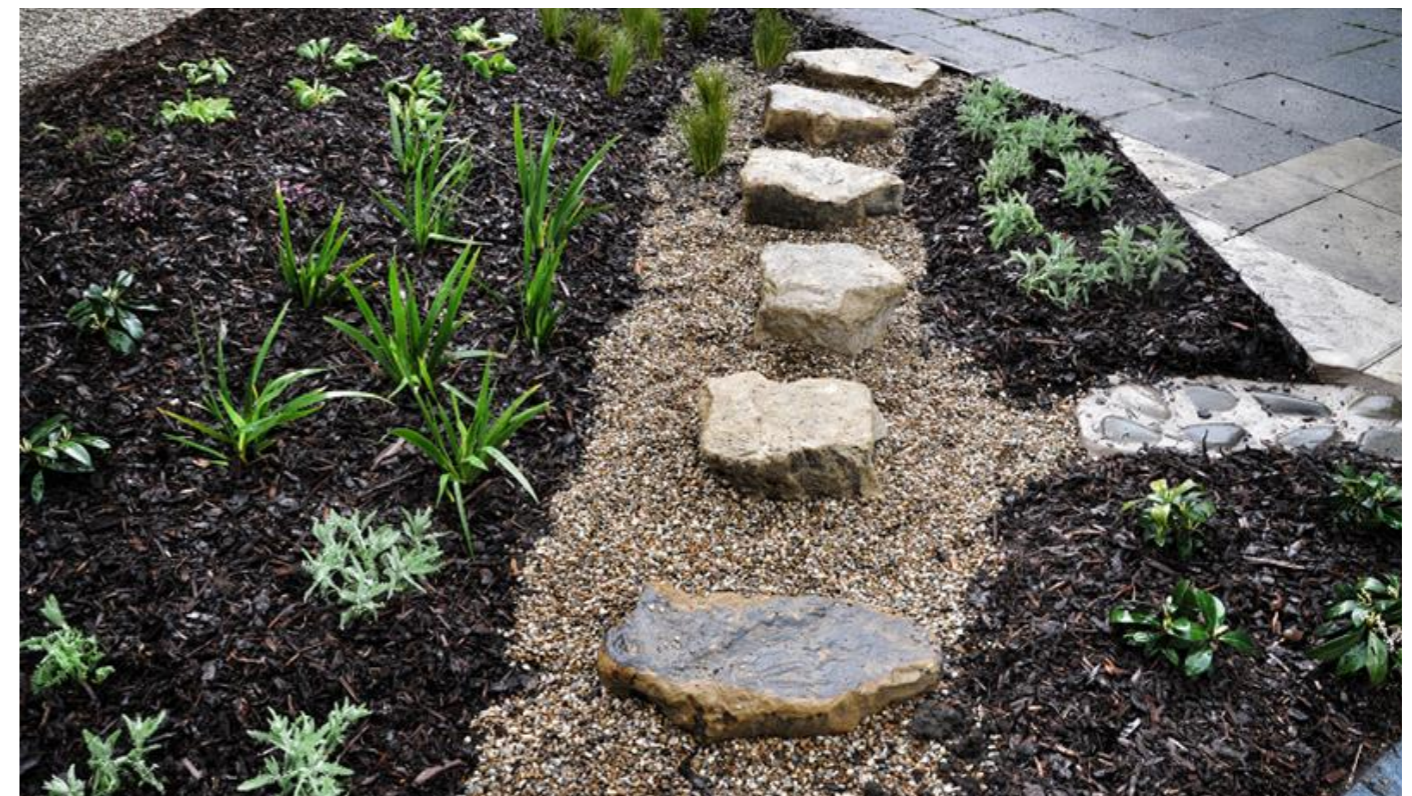
Figure 36. SUDs - Planting bed and permeable paving at Moorland Junior School, Sale Image from: https://www.susdrain.org/case-studies/pdfs/suds_awards/025_18_04_30_susdrain_suds_awards_moorlands_junior_school_suds_sale.pdf
